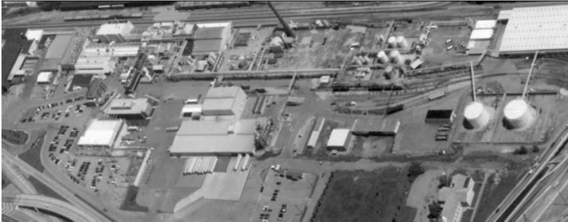
Photo: Rohm and Haas' Knoxville, TN plant
